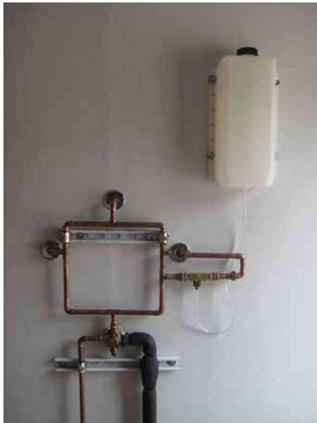
Mechanical room view of bay valves and soap system
