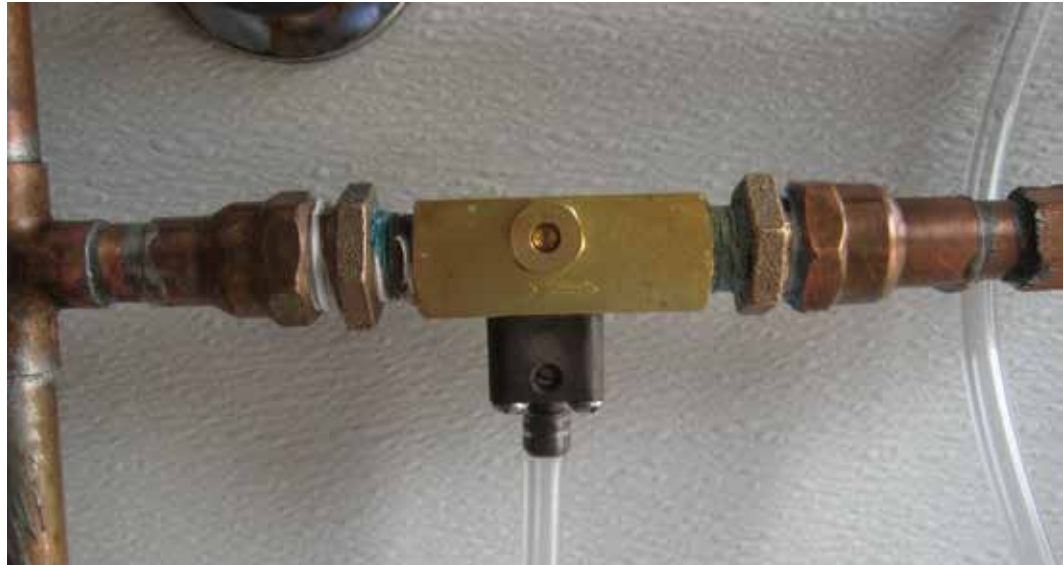
Soap injector valve with adjustment screws
